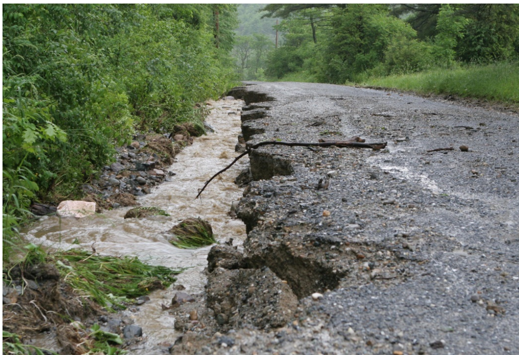
Stormwater degrades a Monkton road
