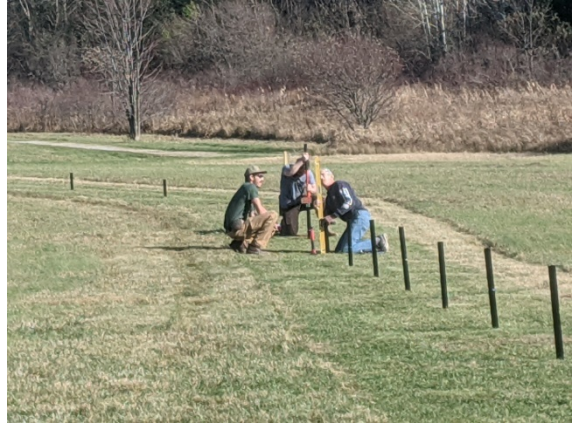
Red School House Contracting: Building the fence
