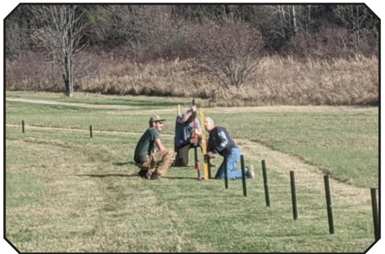
Red School House Contracting: Building the Fence
