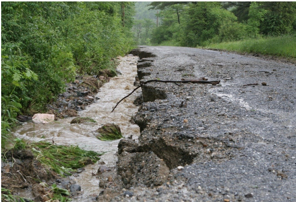
Stormwater degrades a Monkton road
