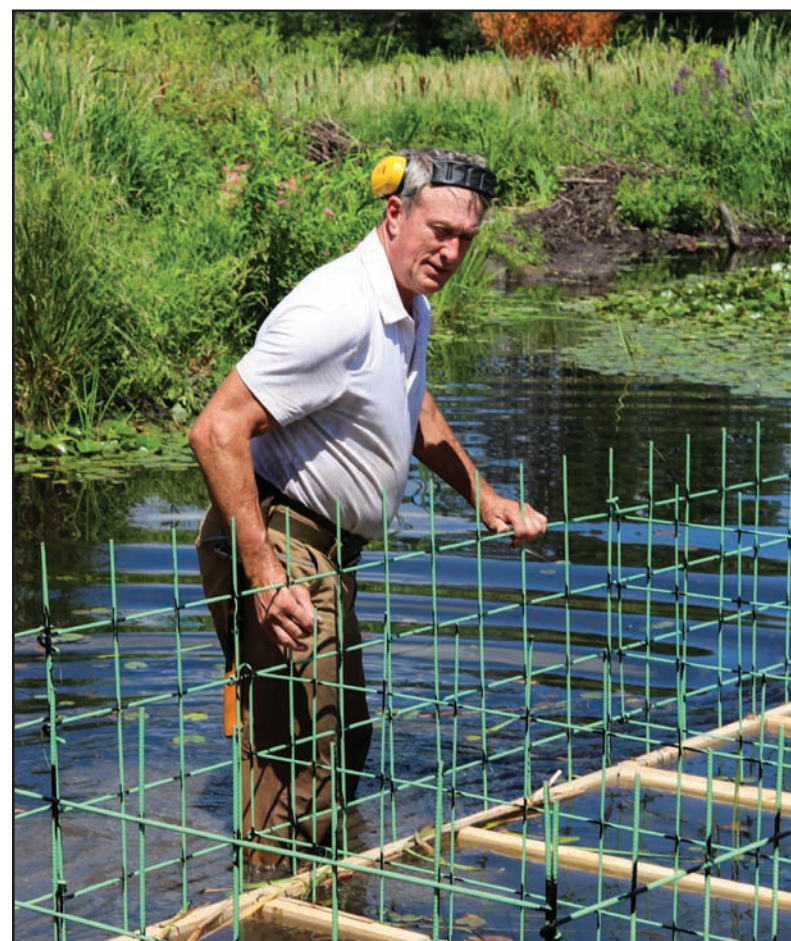
SKIP LISLE FLOATS a Square Fence Filter out onto Monkton Pond last month. The device, part of a system Lisle invented called the “Beaver Deceiver,” will prevent beaver dams from raising water levels enough to flood nearby roads and houses.
